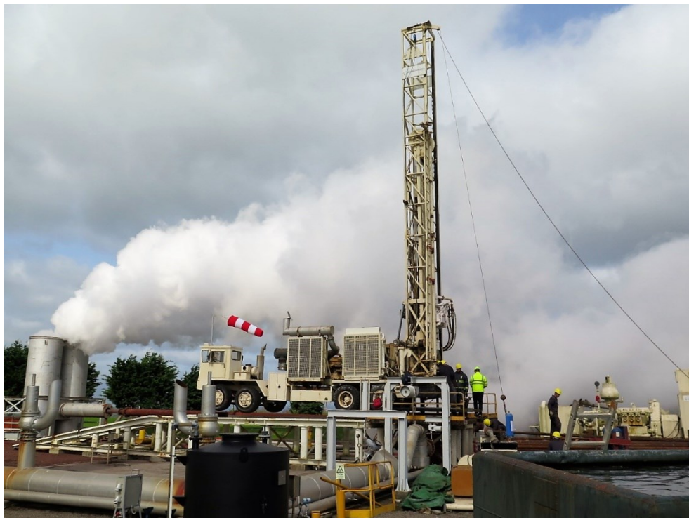
Figure 13: Mechanical reaming while discharging at well PV8 (March-2017)
