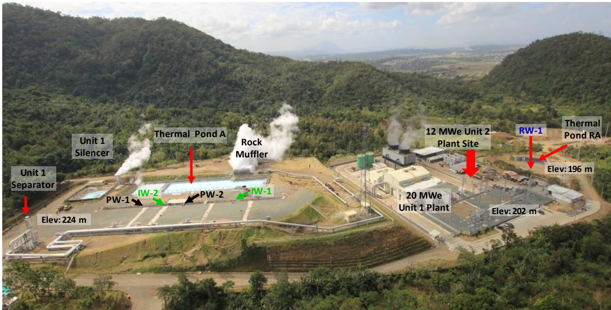
Figure 3: Maibarara field 20 MW steamfield and power plant site where the original reinjection system was designed to reinject the separated hot brine directly into IW-1 and IW-2 (green font). Plant condensates are injected into RW-1 (blue font).
