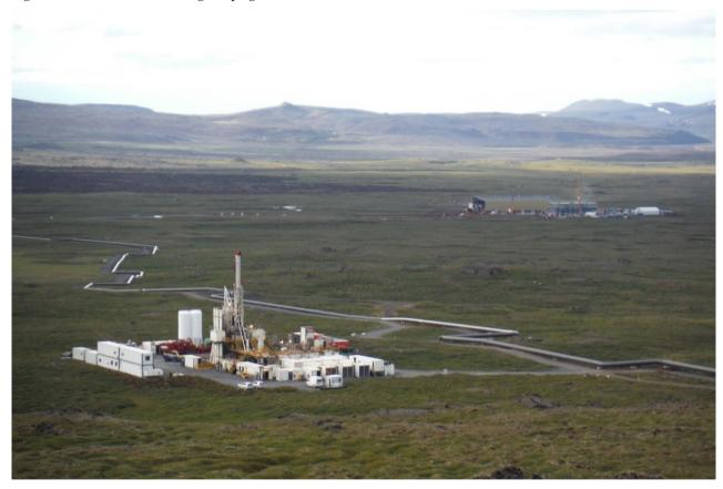
Figure 8: Rig Ódinn on well THR-12 in September 2016. Steam pipes and powerhouse under construction in the background.
