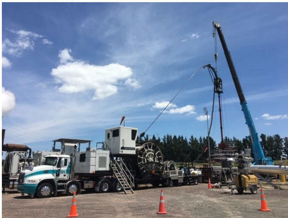
Figure 2: Western Energy live well cleanout operations on a well at Contact Energy's Wairakei Field in New Zealand
