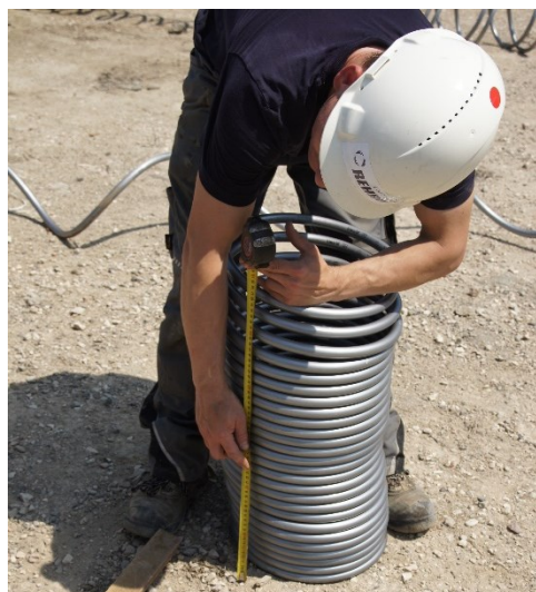
Figure 3: RAUTITAN stable pipe before the extension process.
