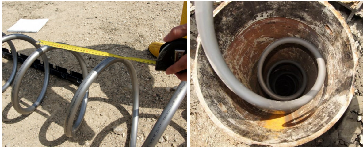
Figure 4: a) No need for retaining bands or other fixations. The new 25 × 3.7 mm stable pipe from REHAU AG+Co retains its geometry after the extension process (left). b) The spiral prototype installed within the ‘enlarged easy drill’ hollow auger segments (right).
