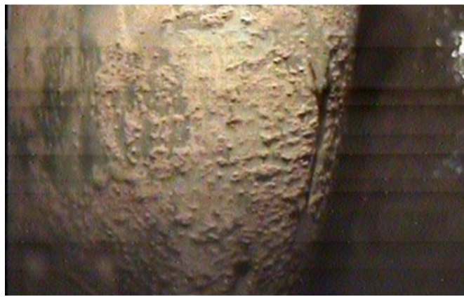
Figure 3. The photo shows the bulge in RN-15 at 140 m (from camera run August 12th, 2016).
