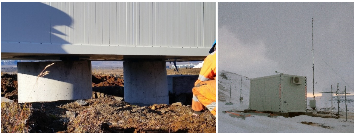
Figure 2: Placing the container for the gravity meters on the concrete pillars at SCGE (left) and the final setup of each gravity station with the hydrometeorological instrumentation installed (e.g., SCGE) (right). (pictures: P. Jousset, K. Erbaş)
