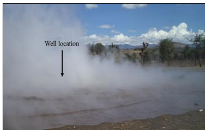
Figure 6. Picture showing the blowout well during drilling in May 2014.
