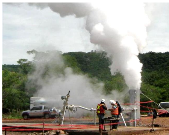
Figure 3 A flow test of 1,300 m deep angled slimhole in Mita, Guatemala. Final hole size was HQ (100 mm). Production was about 1 MW e .
