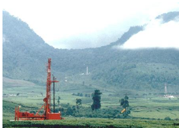
Figure 11: Combined slimhole (orange rig in foreground) and conventional well drilling (white rigs in background) approach used at Wayang Windu, Indonesia in 1996.
