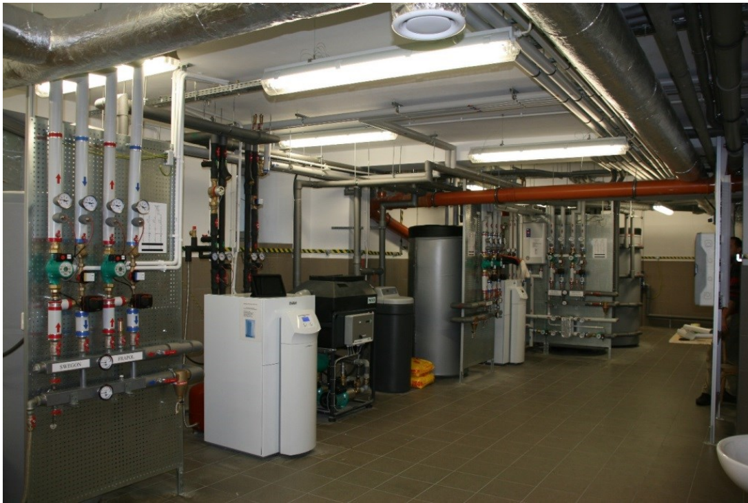
Figure 2: The view on a boiler room with installed heat pumps.
