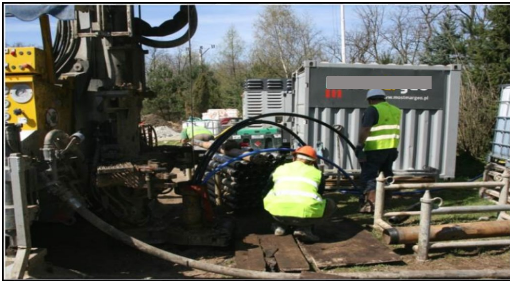
Figure 7: Drillings for borehole heat exchangers in the Centre
