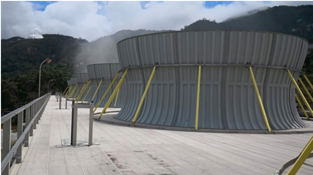
Figure 4. The “enhanced support system” includes a steel support ring at about two-thirds the height of the fan stack and a stainless lower ring spread out from the base of the fan cylinder. The struts are square FRP pultrusion tubes connecting to the SS ring.
