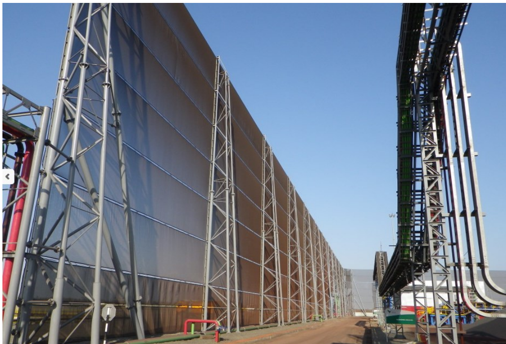
Figure 6: Wind dust control in Oman 30m (100ft) x 3150m (10,300ft). ( http://weathersolve.com ).
