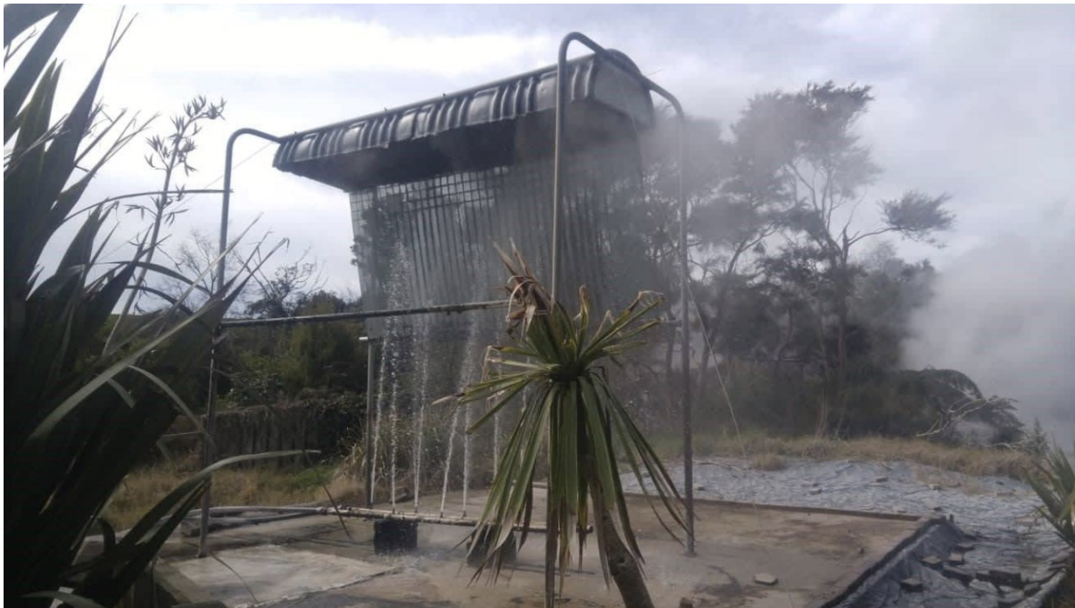
Figure 9. The open air shower cooling system at the Waikite Valley thermal pools.
