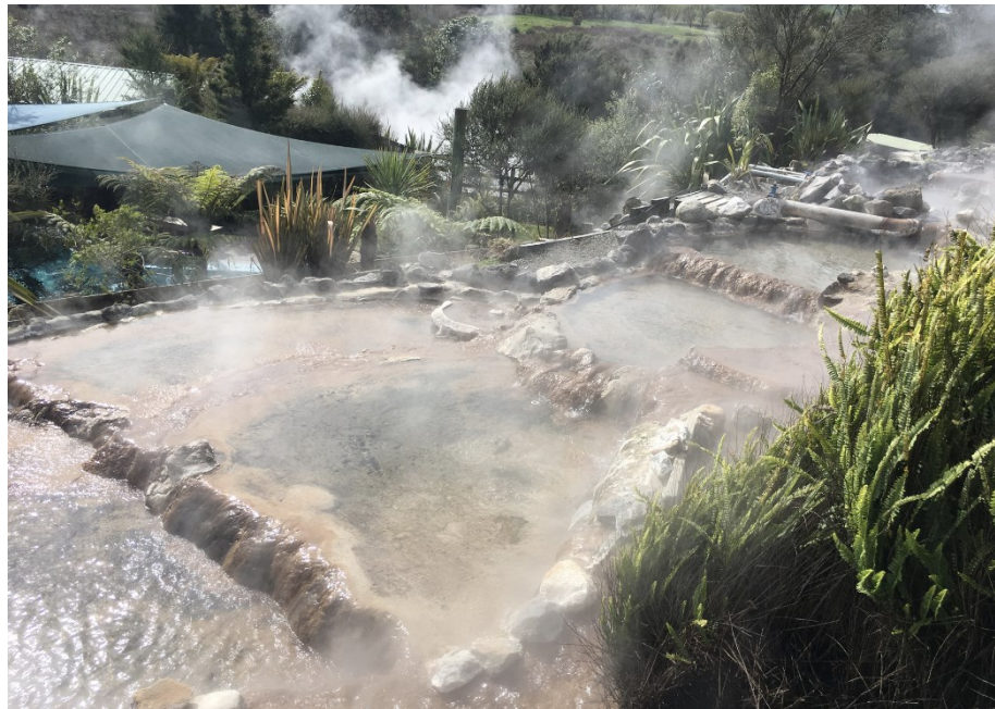
Figure 10. The sequence of smaller (man-made) cascade terraces designed for cooling before the thermal pools.
