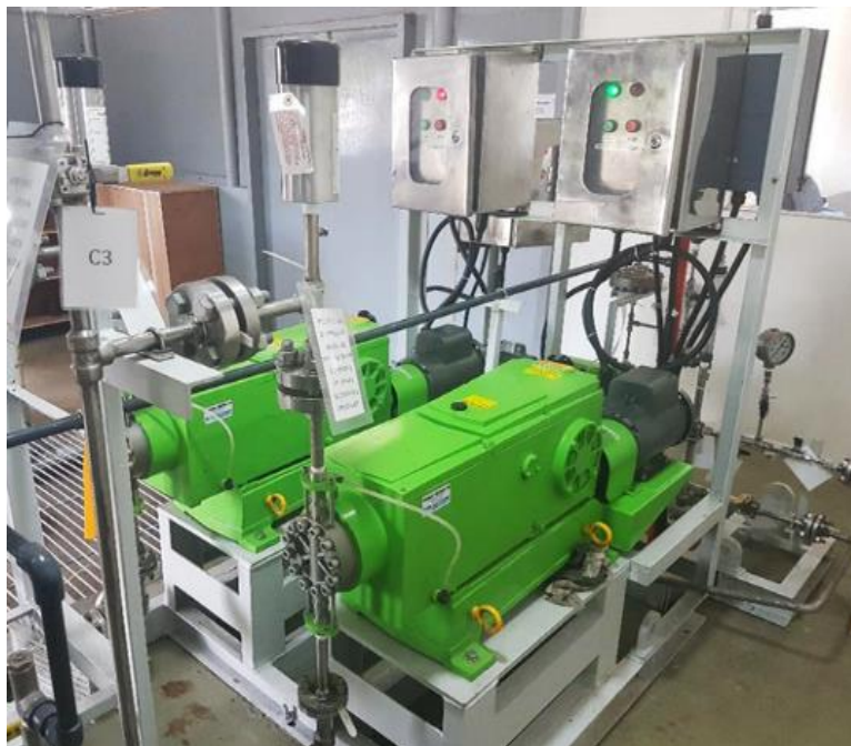
Figure 6: Pulsafeeder 7660-S-E used as injector pumps for the FMS. Two (2) units are installed to serve as a 100% back-up.
