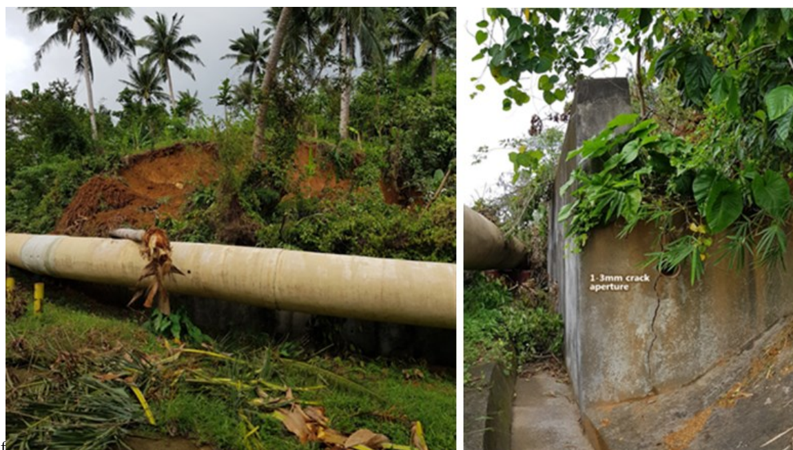
Figure 1. Retaining wall protected the pipeline from landslide in the Tiwi Matalibong area.
