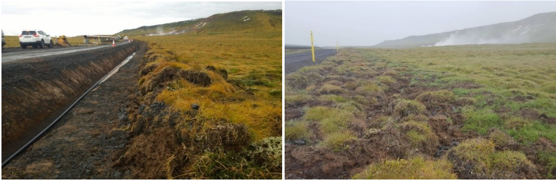
Figure 1: Left: Vegetation cover is removed during constructions at Hellisheiði Power Plant and retained on the edge of a pipe ditch. Right: Native turfs one year after transplant on top of the same pipe ditch as in the picture on left. Photos: Magnea Magnusdottir
