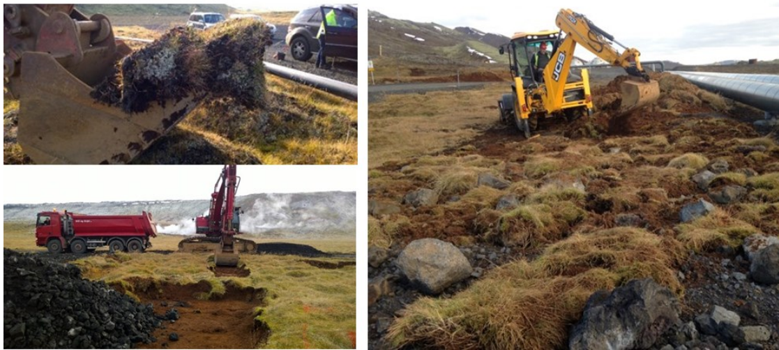
Figure 2: Vegetation cover removed during road constructions at Hellisheiði Power plant, transferred on a truck and transplanted on the edge of a drilling platform. Photos: Magnea Magnusdottir
