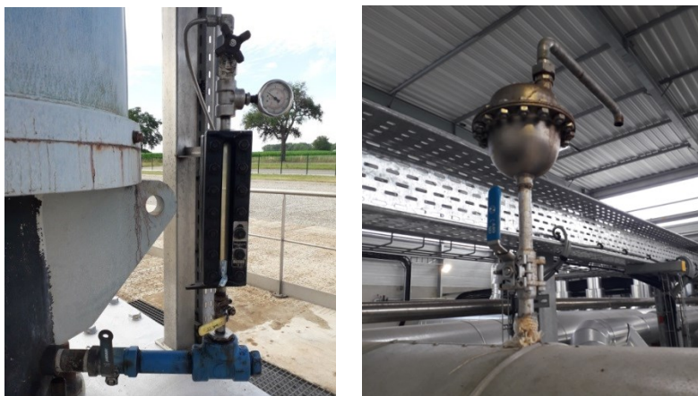
Figure 3: View of the gas sample assembly designed by the downhole pump supplier and of a venting valve on the piping installation (source ES).
