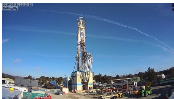
Figure 1: HAS Innova drilling rig on Borehole UD1 at United Downs Cornwall. February 2019
