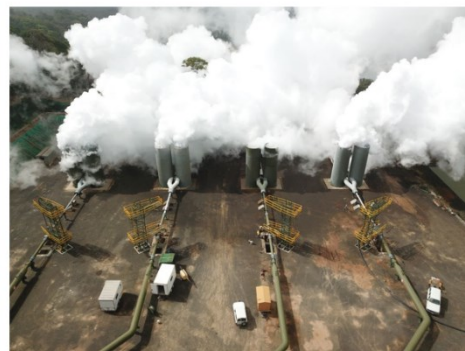
Figure 8: Pailas II Unit, a 55 MWe flash plant installed by 2019 at the Las Pailas Geothermal Field.
