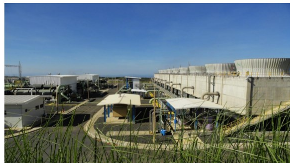
Figure 7: Pailas I Unit, a 42.5 MWe binary plant installed by 2011 at the Pailas Geothermal Field.
