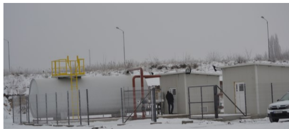
Figure 5. Reinjection well site (storage tank, pump station, and reinjection well shed).
