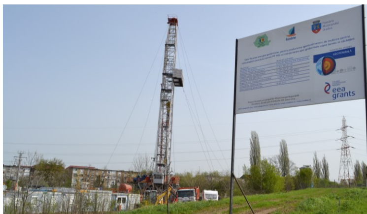
Figure 3. Drilling the reinjection well.
