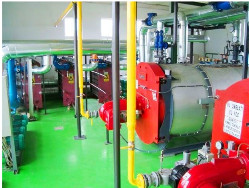
Figure 7: Geothermal heat plant (HX1 and peak load boilers)
