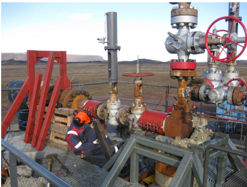
Figure 19: Flow control valves in pair, one with handwheel, the other with hydraulic ram.
