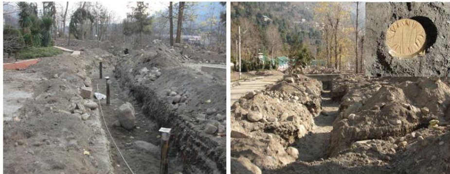
Figure 8: (a) The drilled boreholes as shown by uncut top portion of MS-casing in trench, (b) the top cut view of covered borehole and trench after cutting top portion of the MS-casing (ready for installation of U-bent).
