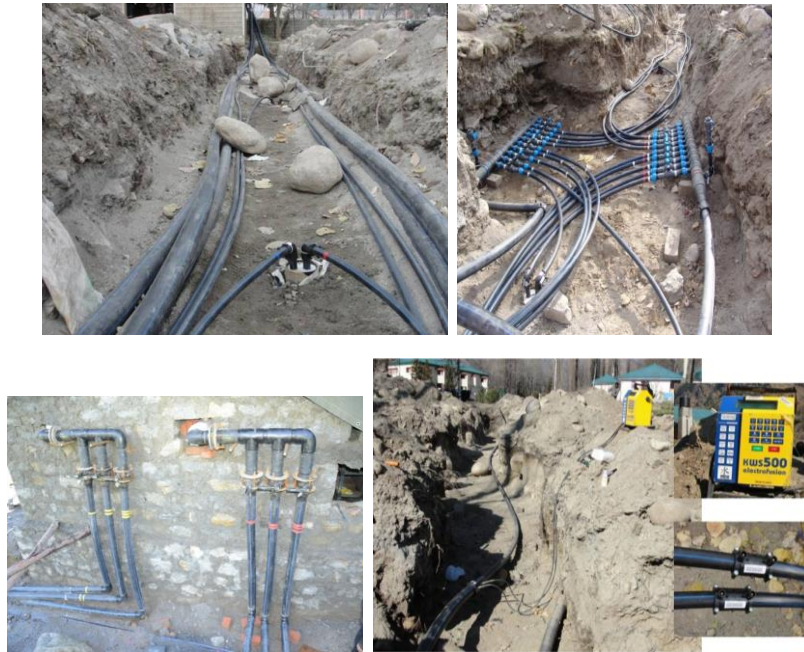
Figure 10: (a) Erected horizontal and vertical loop, (b) connection to manifolds, (c) the header connections (1X3 and 3x1) to GSHP, (d) ongoing onsite electro fusion work of the pipe joints/fittings.
