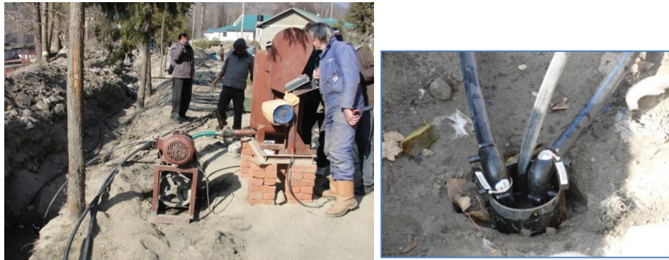
Fig. 12 : Grouting work going on at the project site (a) grout pump, grout paste entering into borehole through a 32 mm pipe.
