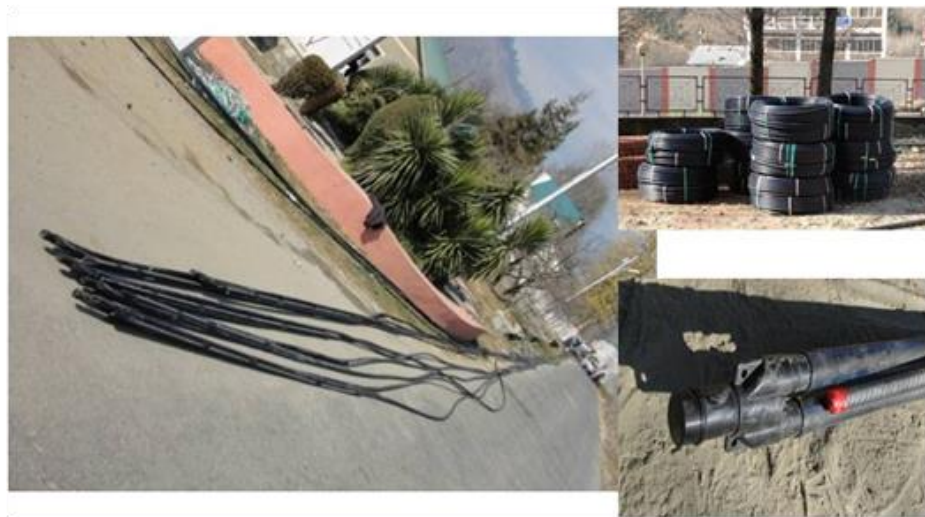
Fig. 9: HDPE U-bent for vertical boreholes installation, top view is the roll of HDPE pipes (U-bent) and bottom view id the end of U-bent.
