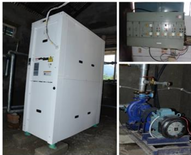
Figure 13: The Ground Source Heat Pump installed at the project site along with its control panel (right side top) and circulating pump (right side bottom).
