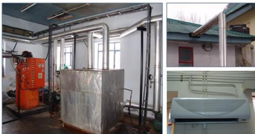
Fig. 14: Performance evaluation of GSHP based space heating system with existing central heating plant connected to the dwellings.
