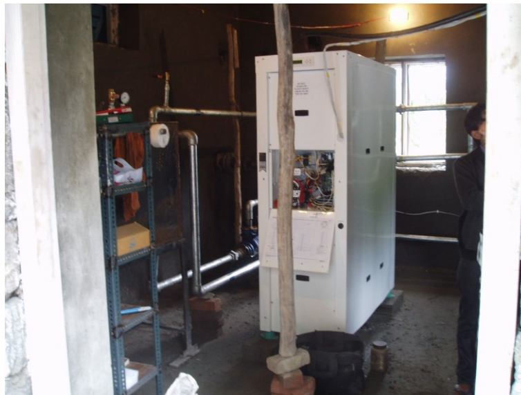
Figure 7: Water Furnace Envision heat pump in plant room.
