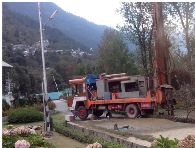
Figure 2: Drilling of the borehole for the thermal response test.
