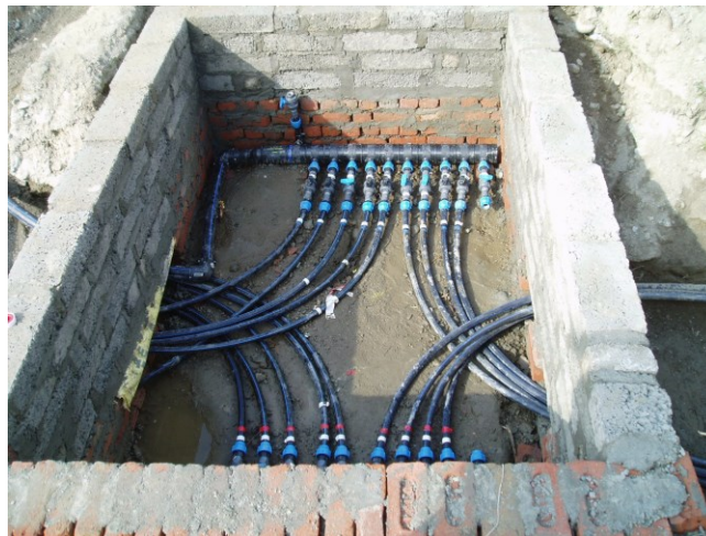
Figure 5: One of three manifold pits, showing manifolds, isolation valves and nine pairs of borehole connections.
