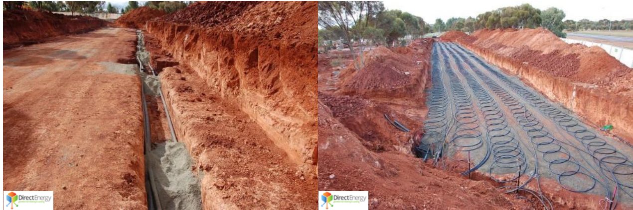
Figure 7: Installation of combined Vertical & Horizontal GHX (44 x 96m + 10 x 25m, 10 x 36m, 10 x 50m Slinky).
