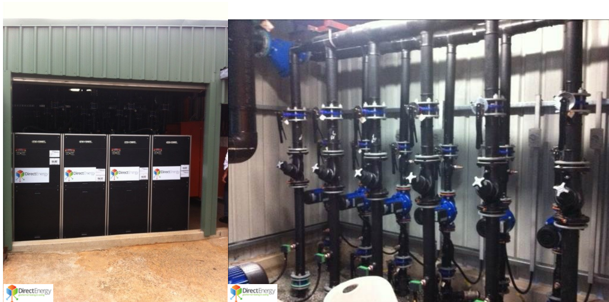
Figure 14: Four GSHPs (left) and 6 pipes leading to GHX (right).
