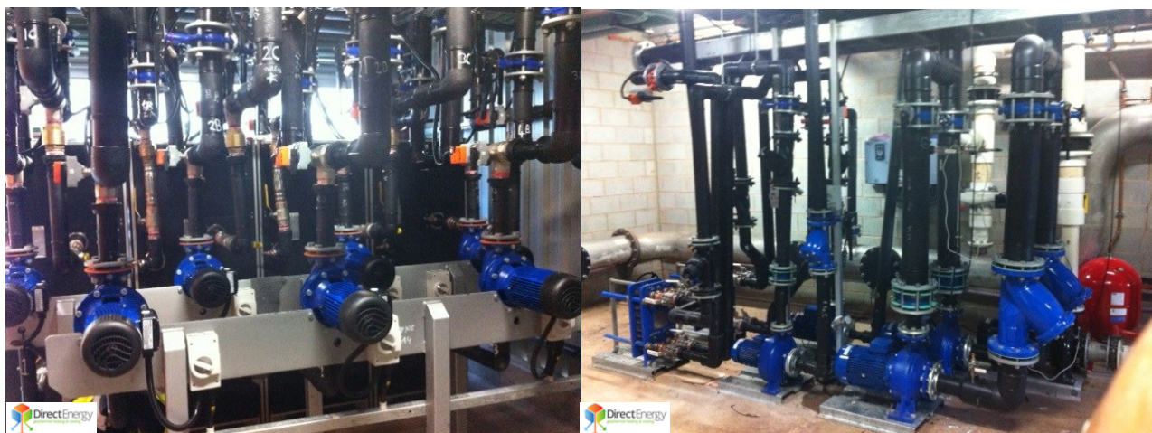
Figure 15: Pumps & Header pipes for GSHPs (left) and Pool Heat Exchanger & Pumps (right).
