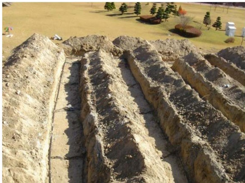
Figure 1: Schematic diagram of GHE array and a photo of the site. The object system is located at the Earthquake Research Center building of KIGAM, Korea.
