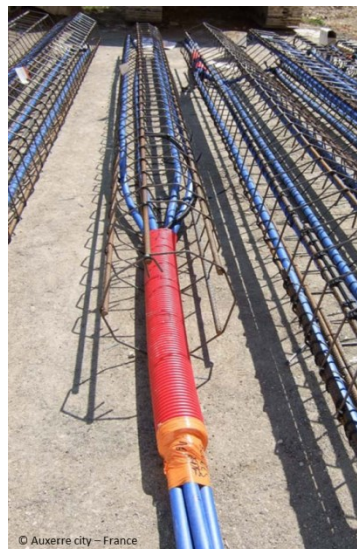
Figure 1: Example of a pile heat exchanger (PHE) before installation in ground (with the courtesy of Auxerre city – France)
