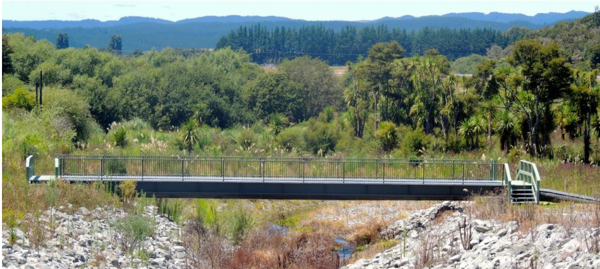
Figure 6: Reinjection pipeline concealed within pedestrian bridge structure
