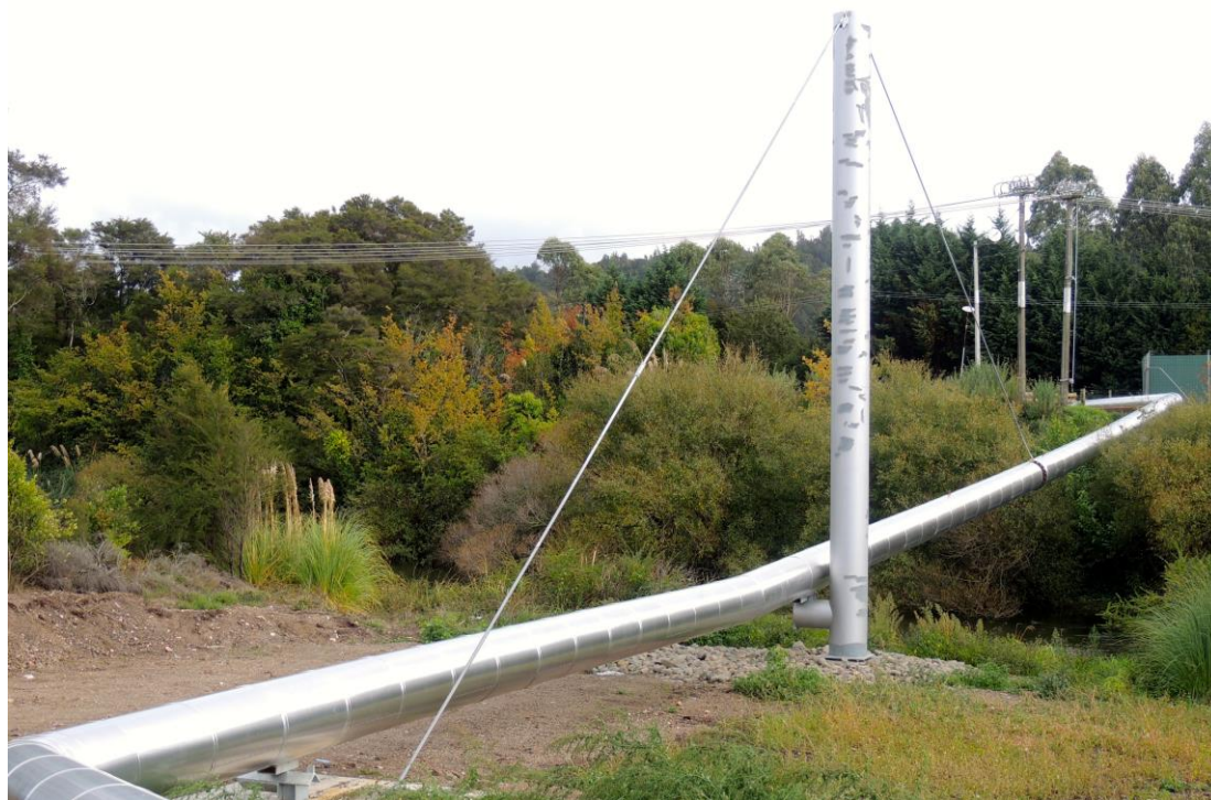
Figure 5: KA30 two-phase pipeline spanning the Tarawera River
