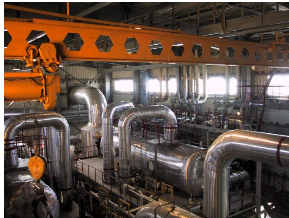
Figure 6: Mutnovsky GeoPP. Primary separators provide MGeoPP with the high-quality steam. (Photo of Svalova V.).
