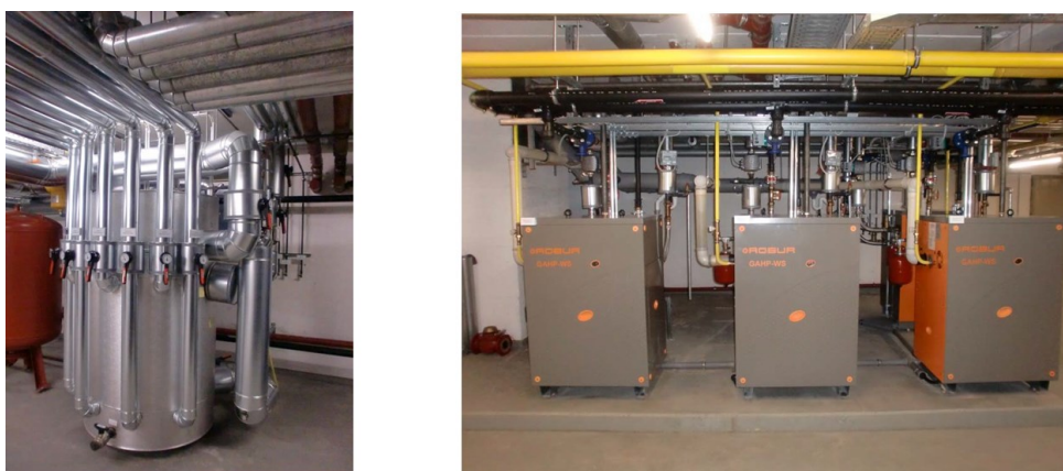
Figure 7: Warm-Water- deflector and heat pumps in the plant room of the school, Bucker (2013)
