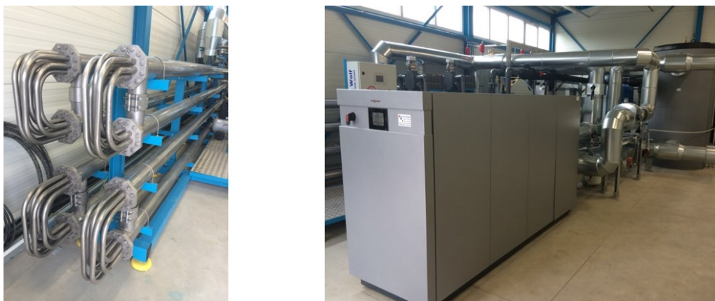
Figure 9: Tube bank heat exchanger and a heat pump at the Erftverband site in Erftstadt.
