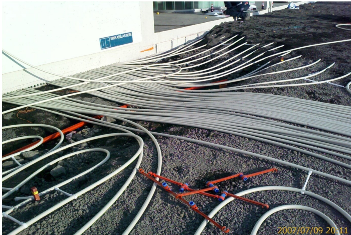
Figure 5.Snow Melting Implementation in Iceland
