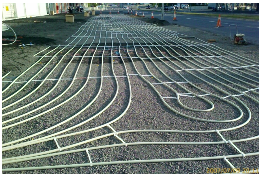
Figure 1. Snow Melting Implementation in Iceland
