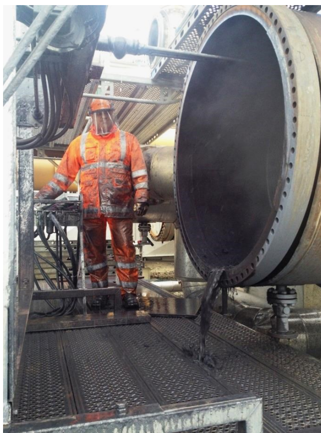
Figure 14: Manual cleaning of the OEC heat exchangers
