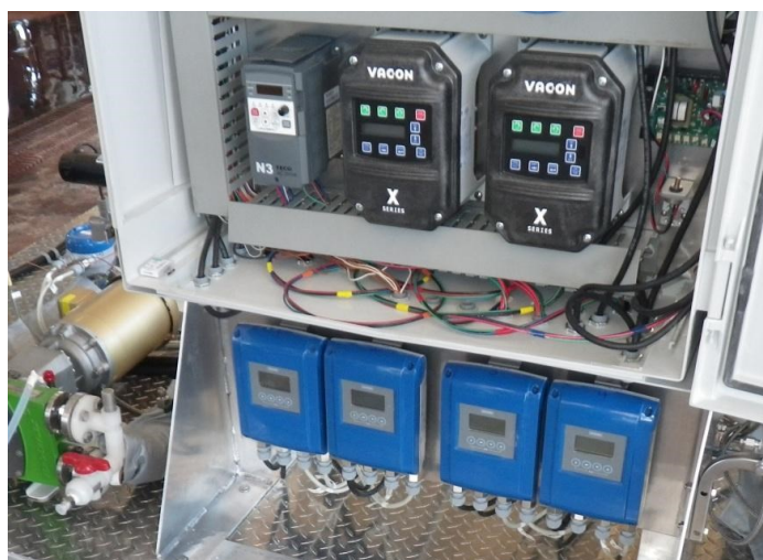
Figure 3: HUV and Packed-Bed Test Skid Flowmeters and Pump Control
