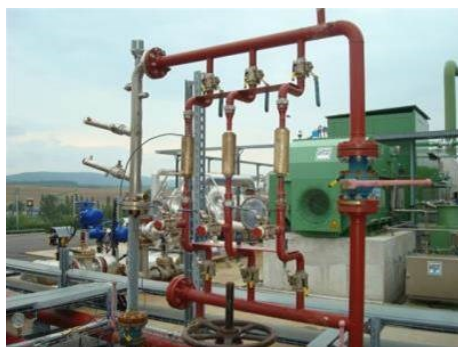
Figure 6: Low temperature skid (LTS) is located downstream of the heat exchanger before injection well GPK-3 at the reinjection side of the geothermal loop at Soultz. After Scheiber et al., (2013a).
