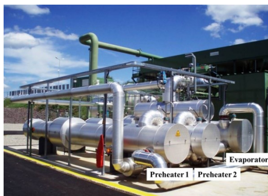
Figure 1: ORC tubular heat exchanger system of the Soultz geothermal power plant: ORC Evaporator, Preheater 1 and Preheater 2, (Picture: GEIE).
