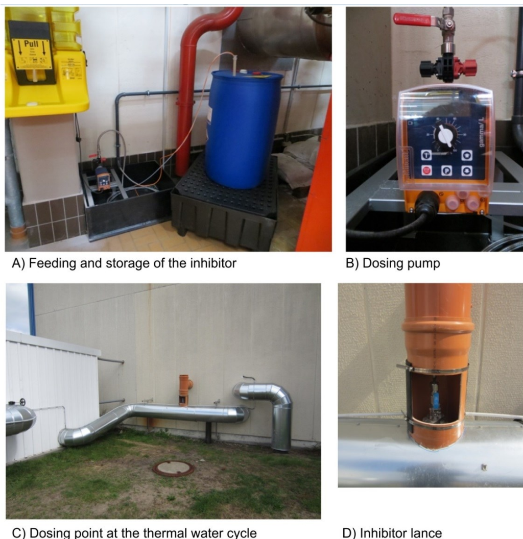
Figure 8: Installations for the inhibitor injection.
