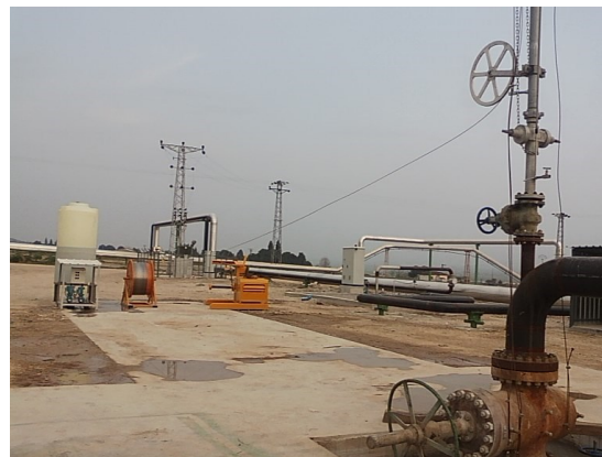
Figure 2: Scale inhibitor system at production well in a geothermal field (Photo: Kizildere GPP-Turkey)
