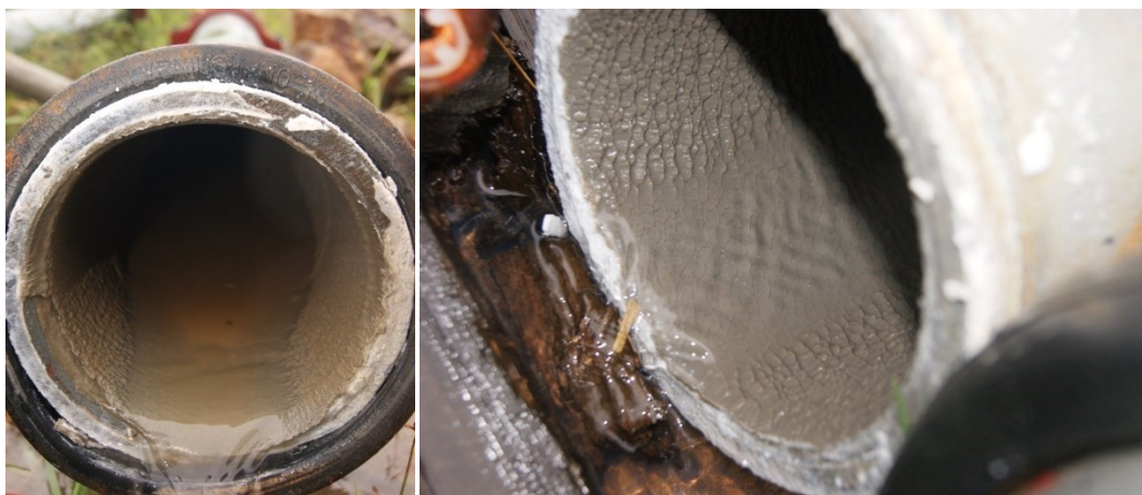
Figure 6: Inspected alvenius lines after increased GSX dosing to 8ppm
