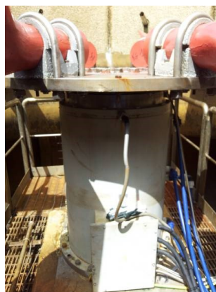
Figure 5 PM Motor installed within the Vallesecolo power station
