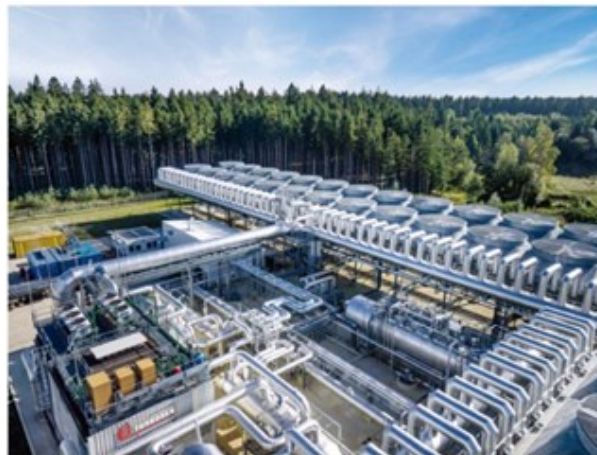
Figure 16 Existing binary plant in Germany designed by Turboden (MHI group company)
