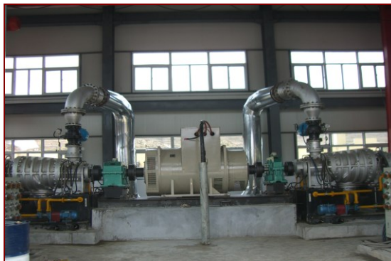
Figure 1: A 1MW screw expander generating unit in YangBaJing geothermal power plant
