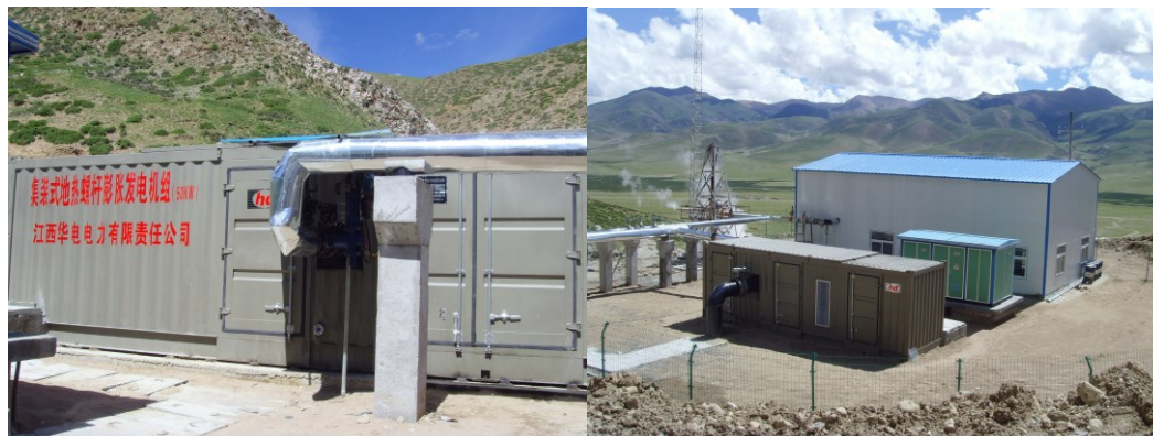
Figure 4: The testing container type of screw expander generating unit in YangYi
