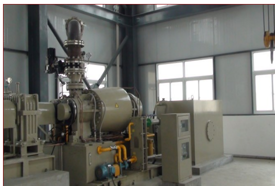
Figure 2: The second screw expander generating unit in YangBaJing geothermal power plant
