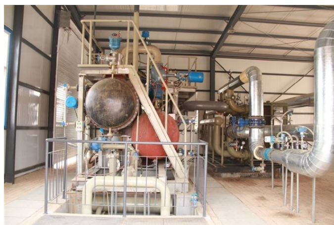
Figure 5: The binary cycle screw expander generating unit in Huabei oilfield
