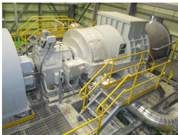
Figure 3: An overview of 20MW Geothermal Steam Turbine
