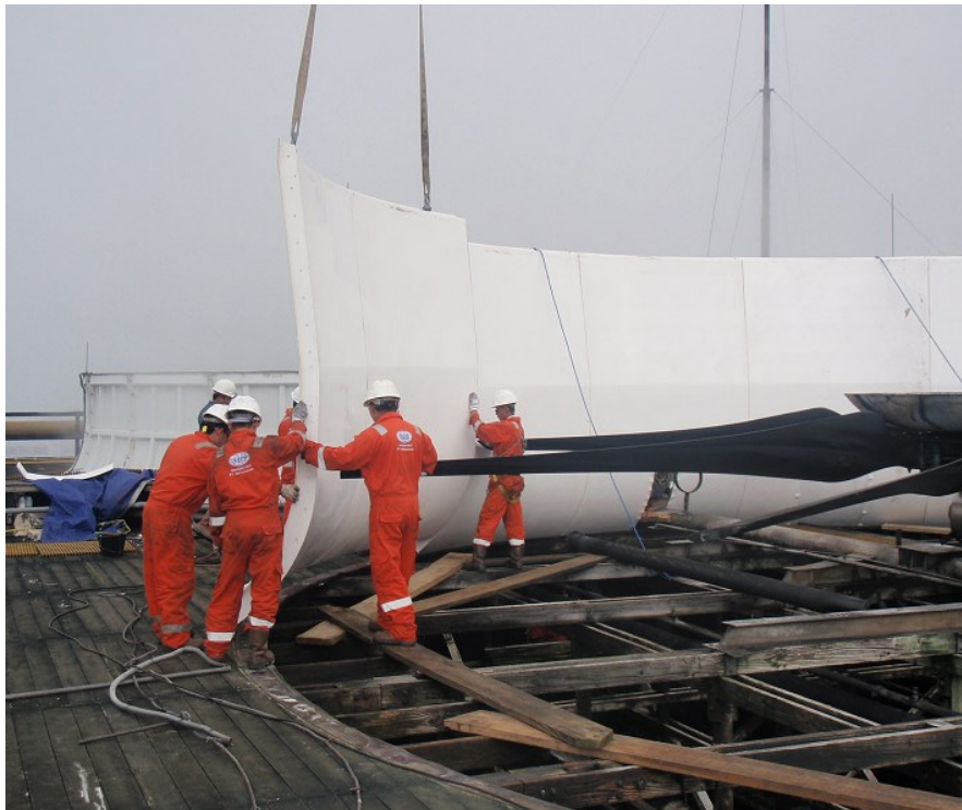
Figure 9: The activity during fan stack modification
