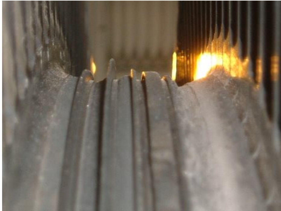
Figure 3: Erosion and missing seal strips found at inter stage between stage 4 and stage 5 Turbine End side.
