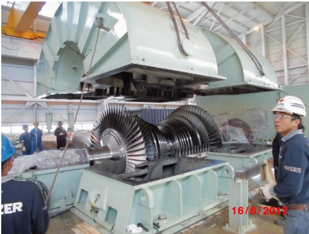
Figure 13: Upper casing installation for top clearance check.
