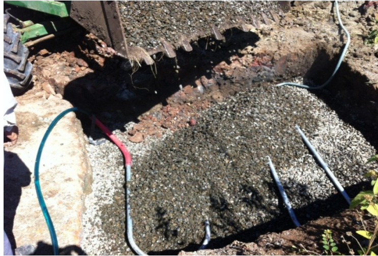
Figure 4: Installation of the heat exchanger J-1 in a pit of 2 m x 2 m x 0.6 m.
