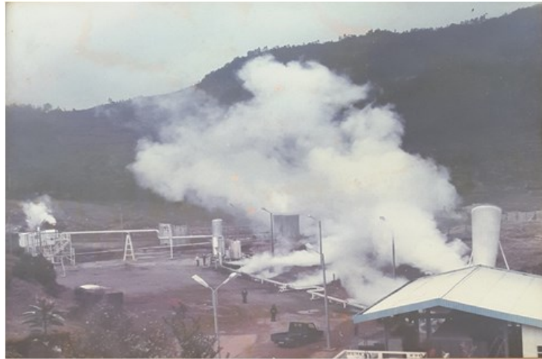
Figure 3: monoblok 250 kW at Dieng field in early year of operation.
