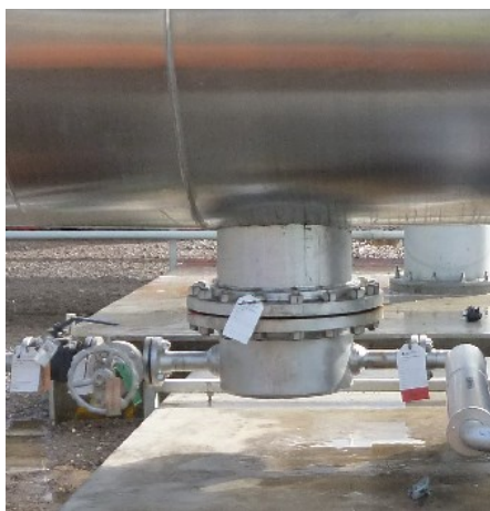
Figure 5 Small drainpot common on many new steam pipelines. Proven as ineffective at removing pipeline condensate.
