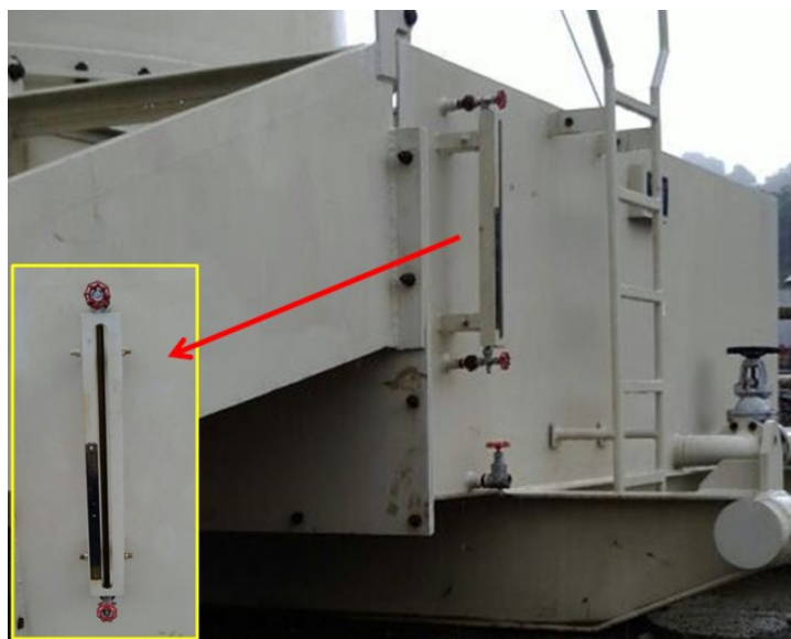
Figure 8. Simple measurement set with U-pipe principle to measure the brine water level in the weir box.
