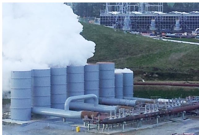
Figure 7: IP+, IP & LP Separated Water Dump Equipment
