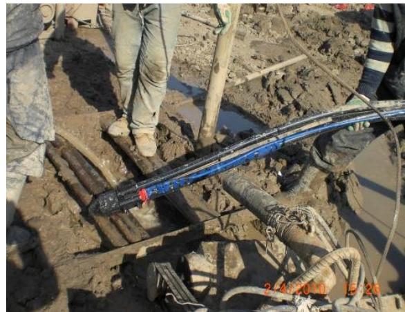
Figure 8: Ground temperature monitoring hole construction and vertical measuring line down into the ground scene graph
