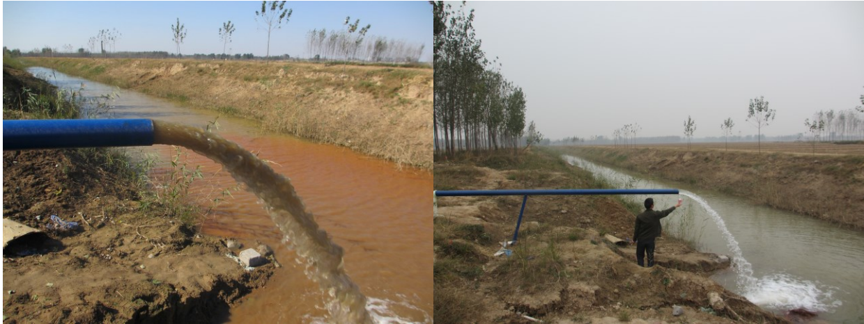
Figure 10: Re-pumping during the reinjection until the re-pumped water to be clear and without sand (Left-at the beginning of re-pumping; Right-at the end of re-pumping)
