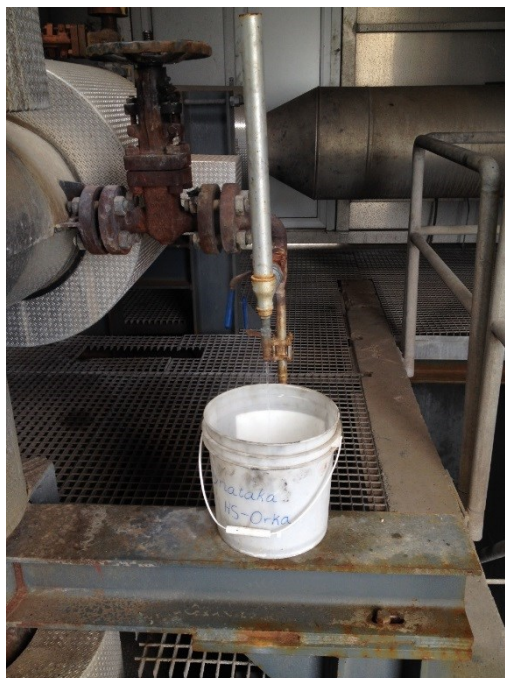
Figure 3: Simple T-shape separator to collect brine samples. The bucket collects excess liquid during washout prior sampling.
